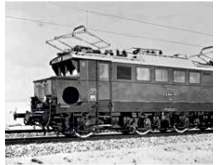
1938 First locomotive using multianode mercury-arc rectifiers from BBC Mannheim, Germany
